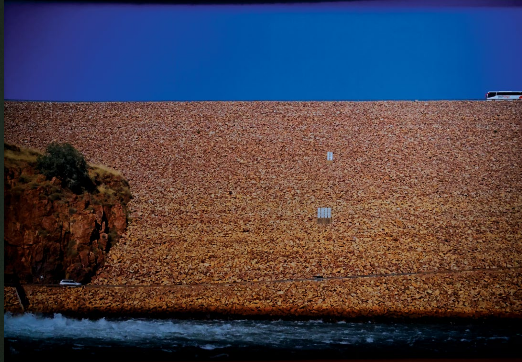
'Faith in a Pile of Stones.' Alana Hunt. 2018. Digital print of 35 mm film photograph, wooden structure, 240 x 360 cm. Courtesy of Diriyah Biennale Foundation .
